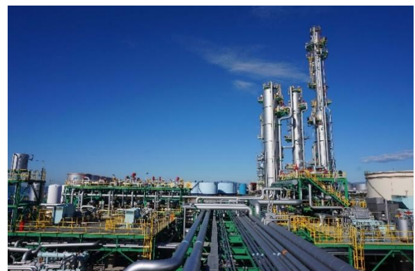
Tomakomai CCS Demonstration Project Center
