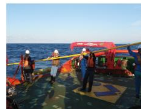
Lowering streamer cable into the sea
