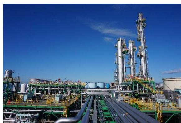
Tomakomai CCS Demonstration Project Center
