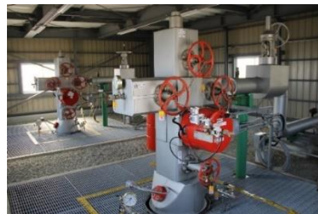
Heads of injection wells
